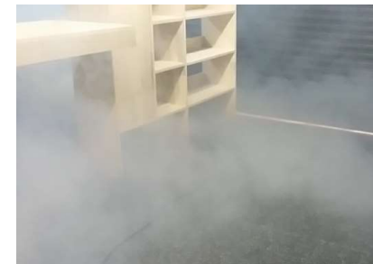
Smoke indicating the airflow. Fresh air being diffuse by the integrated diffusers.
