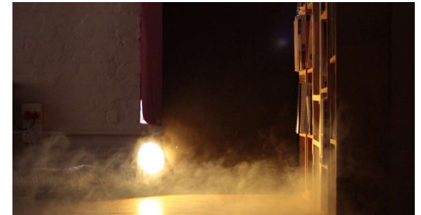
1. Airflow from bookshelf diffuser. Cooler air flowing low to the ground.
